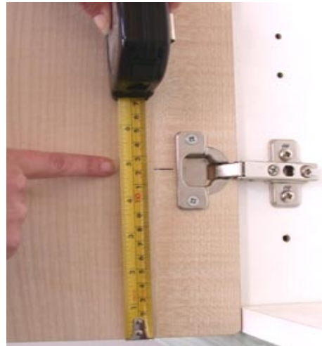
Measure Bottom Hole CENTRE
